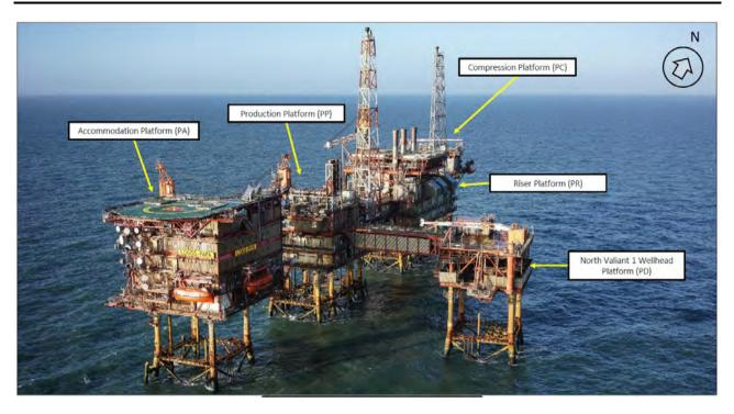
Figure 2-1 Overview of the LOGGS platform captured by UAV
